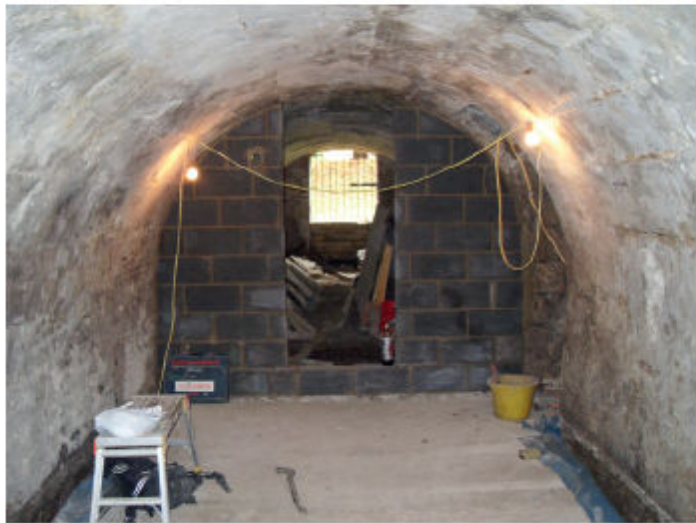
A basement fitted with an ADD waterproofing system
