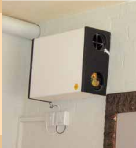
➤ Examples of positive pressure units installed by specialist contractors
