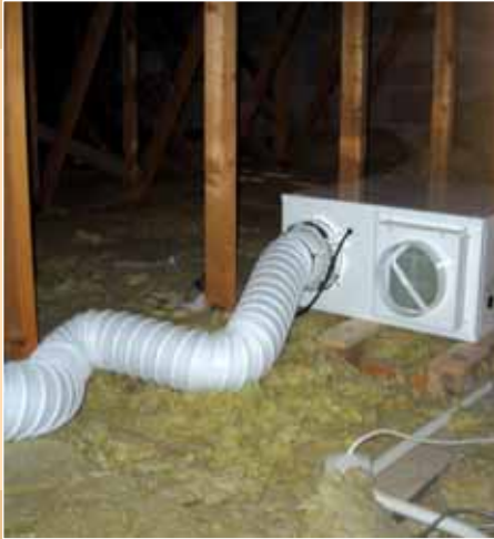
➤ Examples of positive pressure units installed by specialist contractors
