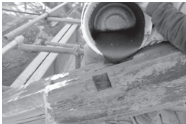
Figure 4. Pouring resin
