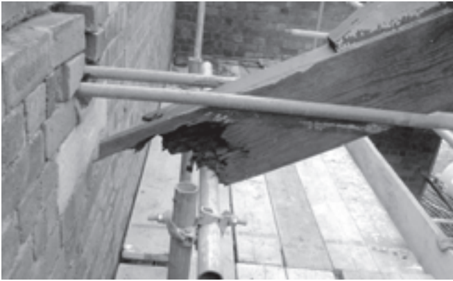
Figure 2. Decayed timber
