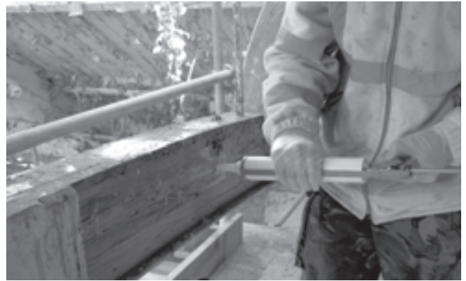
Figure 3. Injecting resin
