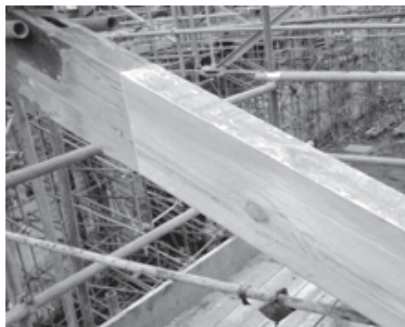
Figure 5. Repaired truss
